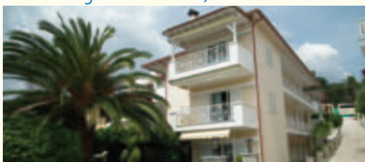
KUĆA PORTO PSAKOU디아 GPS N40.25943/E23.48847
